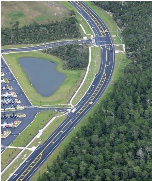
Howland Boulevard improvements.
