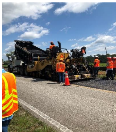
Our Safety Director Steve monitors an A-1 Paving job site.
