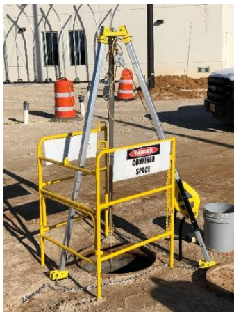
Making sure the fleet is safe while working in a confined space at OCPs #113.
