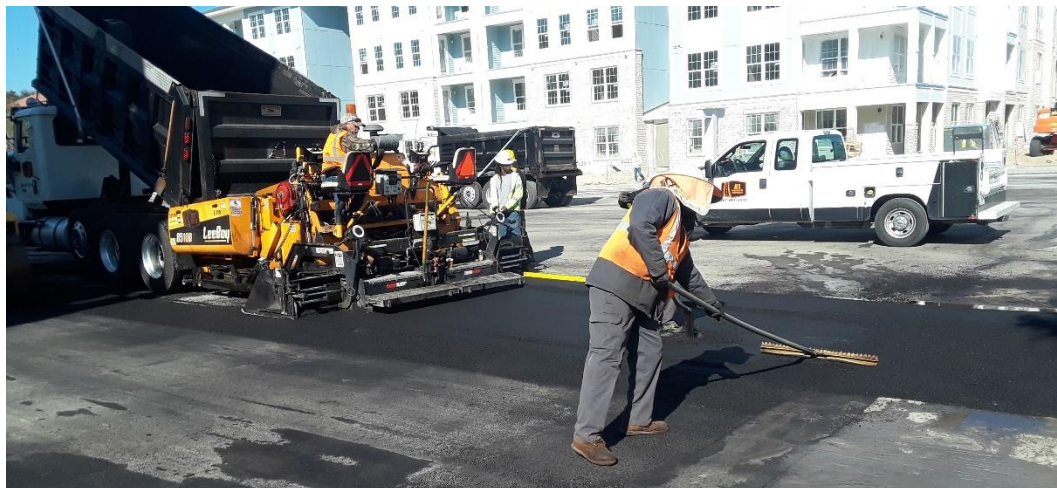
A-1 Paving Project at Integra Apartment Complex.
