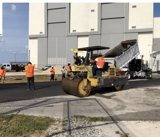
Above and Left: A-1 Crews Paving Safe Haven Road at Kennedy Space Center.
